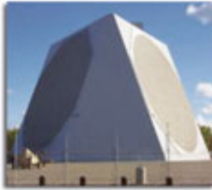
This 27-meter-high radar facility, reminiscent of a fly's eye, scans the sky above northern Alaska and is used as an early warning system against ballistic missiles.
