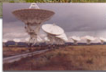
Each of the antennae in the picture weighs 212 tons, and are as high as a 10-storey building and measure at least 25 meters across.
