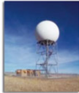
Air radar used to identify powerful storms and track their movements.
